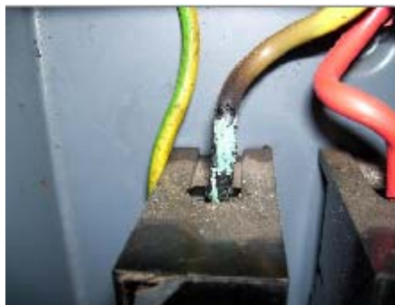
Figure 17. Burnt Wire Min. Possible Fine: $2,000
