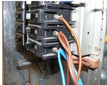
Figure 19. 1 wire per terminal (NEC 110-14a)
