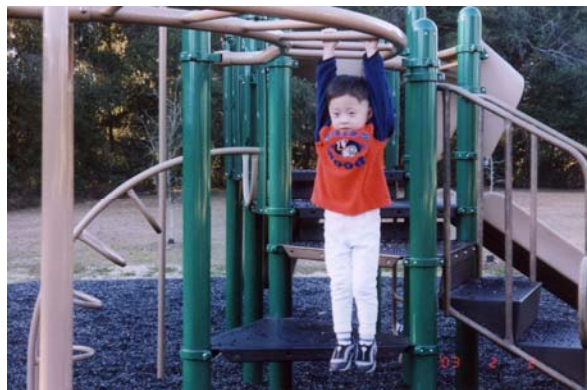
Figure 10. Modern composite play structures are built lower to the ground and covered with a protective surface that limits injury from a fall.
