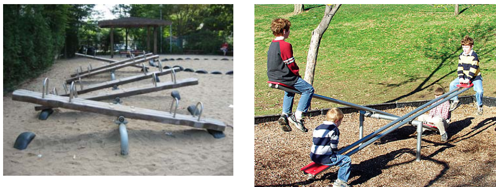
Figure 12. Seesaws require a cushioning device under the seat, like a tire or spring, and the maximum height of the seat cannot be more than 60 inches.
