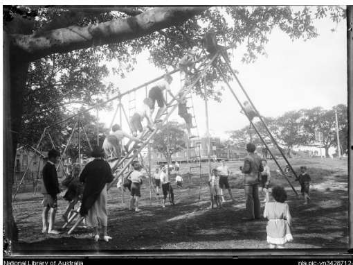
Figure 7. A typical climber from the 1930's presented a high fall risk for users.
