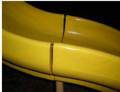
Figure 5. There should be no gaps or openings the length of the slide that could catch clothing or drawstrings.
