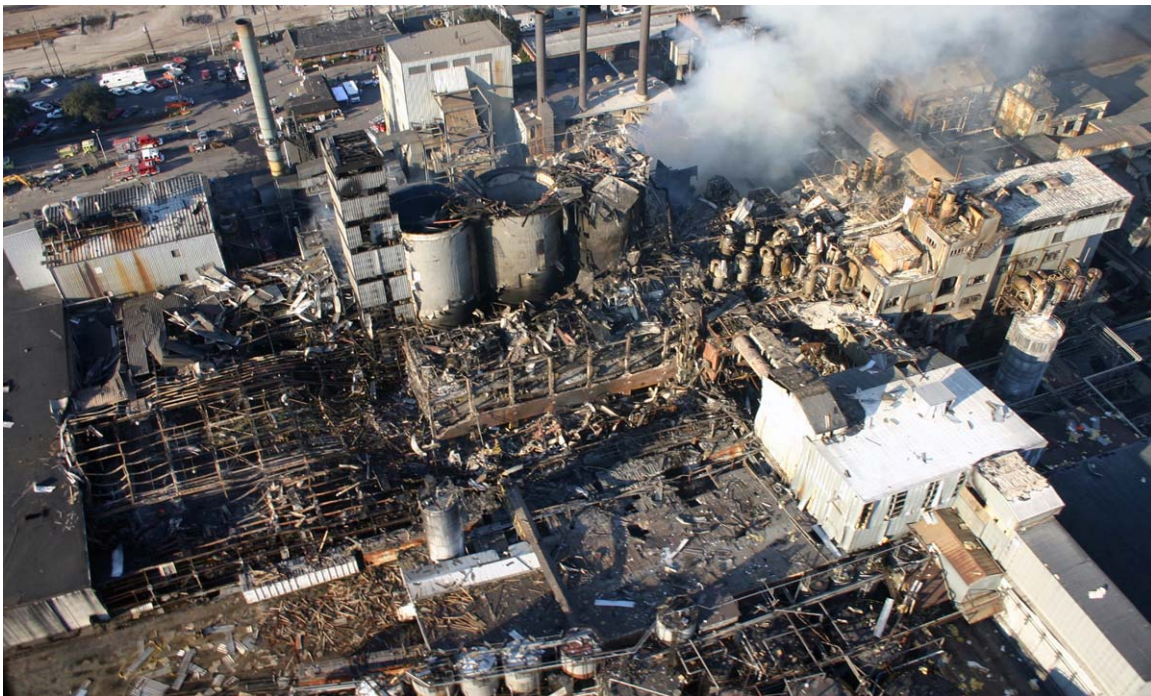
Exhibit 1. Imperial Sugar Refinery's Savannah facility after the explosion. Thirteen workers died, and 39 were injured in this incident. Dust accumulations far exceeded NFPA's recommended limits. (Photo courtesy U.S. Chemical Safety and Hazard Investigation Board.)
