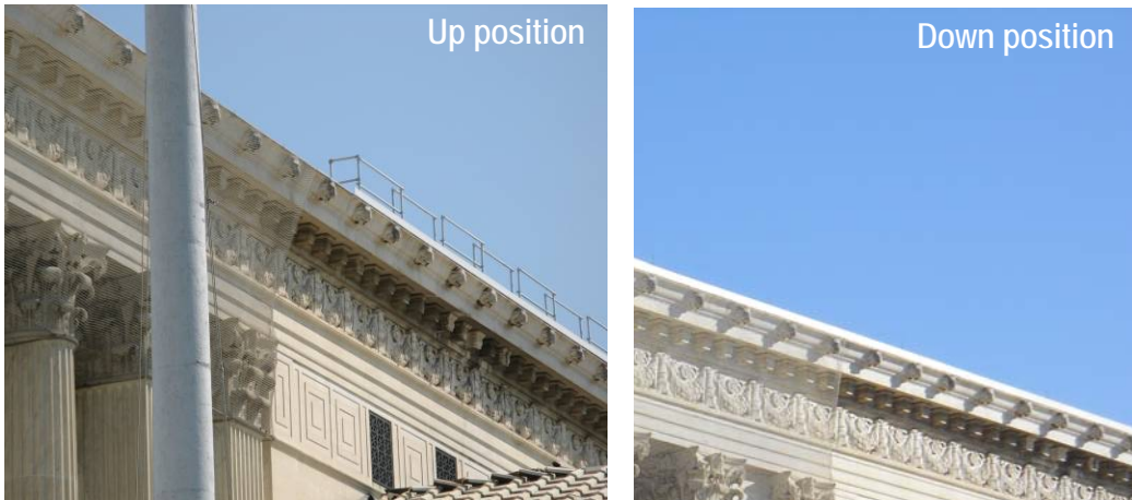
Exhibit 3. To maintain the building's aesthetic and historic value, the new guardrail on the roof of the Supreme Court Building folds down when not in use.
