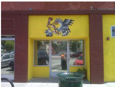
Figures 1: Kindergarten classroom located in former retail location.
