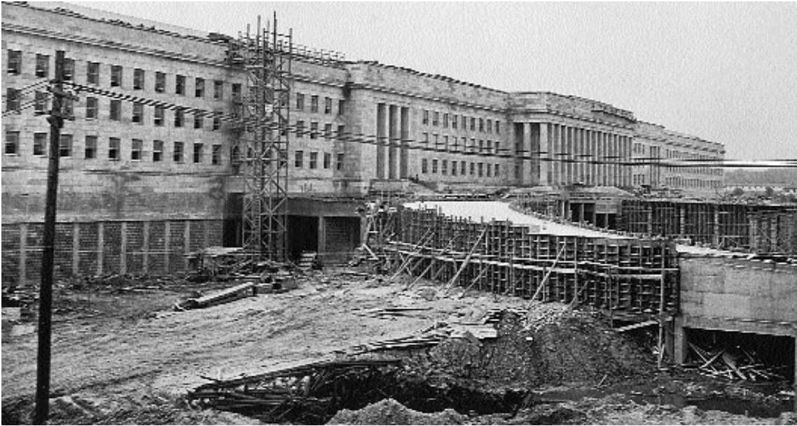
Fig. No. 2: The Pentagon under construction.
