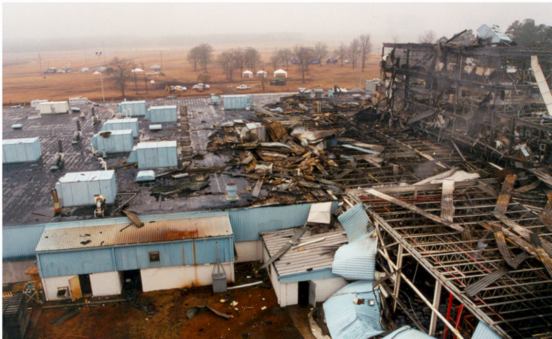
Exhibit 2. West Pharmaceutical Services, Kinston, NC, January 29, 2003. Six people lost their lives, and 38 were injured. Photo courtesy US Chemical Safety and Hazard Investigation Board.
