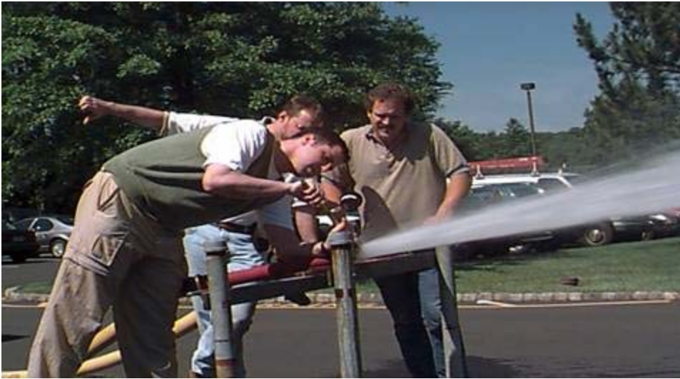
Exhibit 8. Testing Flowmeter by Connecting Hoses to Pump
