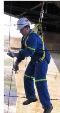
Figure 3 Height of worker (D-ring to toes) at Fall Arrest is nominally 6 ft (1.8m)
