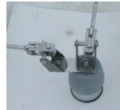
Figure 7 Force Management Anchors add a lot of sag
