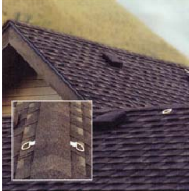
Exhibit 3. This photo shows residential roof tie-offs. By designing and installing roof tie-offs roofers have a structurally sound anchor to tie off on when working on a residential roof.
