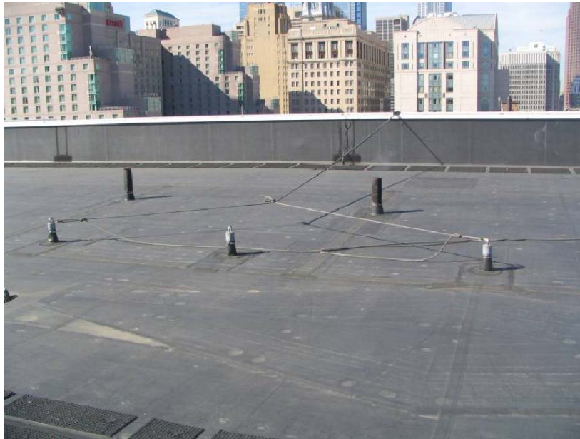
Exhibit 2. This photo shows roof anchorage points. By designing fixed , structurally sound anchorage points workers will have convenient to tie off during construction and future maintenance.
