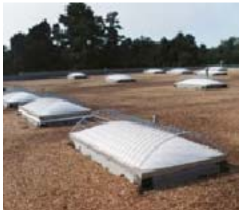
Exhibit 4. Permanent guards over skylights provide protection when working on the roof.
