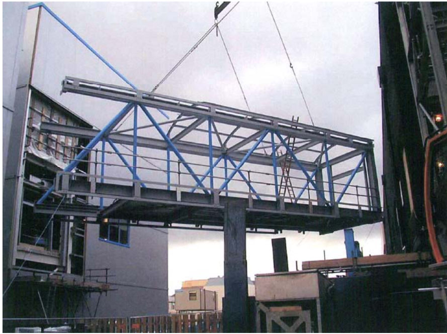
Exhibit 5. This photo shows a pre-fabricated steel structure being lifted into place. By fabricating the structure on the ground less work has to be done at height.
