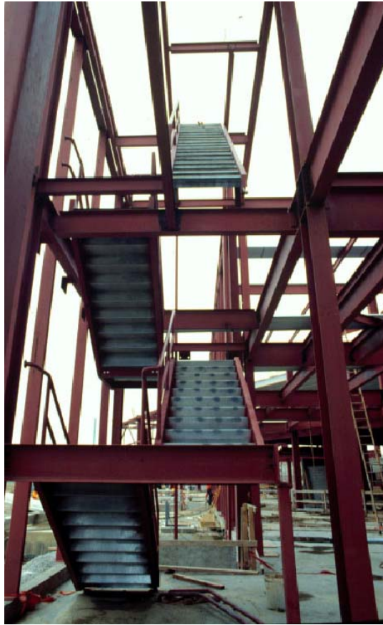
Exhibit 1. This photo shows pre-fabricated stairs. Pre-fabrication of building components reduces the number of work tasks that must be performed above the ground. Pre-fabricated stairs with railings installed early in a project preclude the need for ladders and temporary guardrails.
