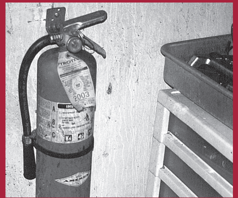
Photo 6 (below): ABC extinguisher found in a commercial kitchen. Employee training should stress the negative impact of using an ABC portable on oil and grease fires.
