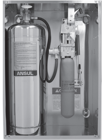
Photo 1: Ansul Automan mechanical release assembly.
