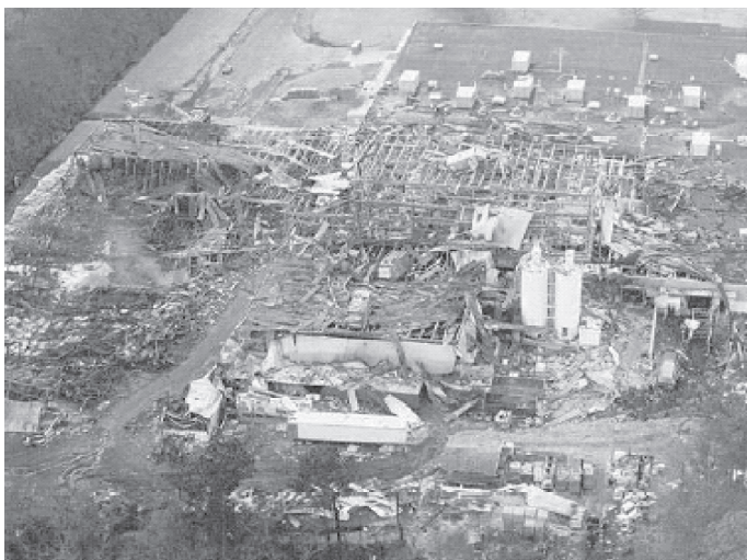
Photo 1: Dust explosion killed six and destroyed West Pharmaceutical plant in Kinston, NC, in January 2003.
