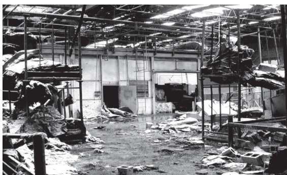
Photo 1: Dust explosion killed six and destroyed West Pharmaceutical plant in Kinston, NC, in January 2003.
