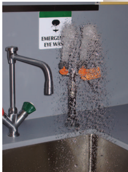
Photo 11 (left): Eyewash at lab sink with proper pressure and flow.
