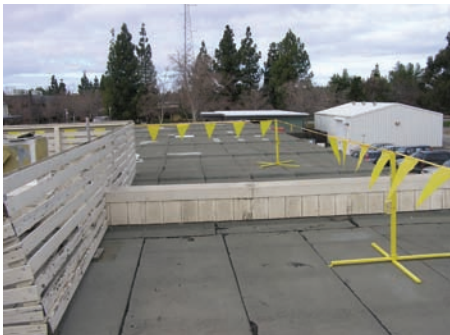
Photos 1 (top) & 2 (bottom): Combined designated area and scaffold stairs.
