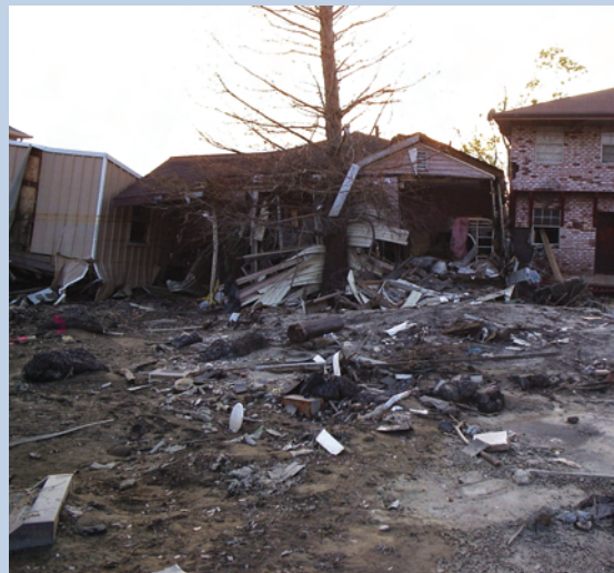
Residential debris, such as that in Orleans Parish, New Orleans, LA, following hurricanes Katrina and Rita had to be hauled to landfills, which created many hazards.
