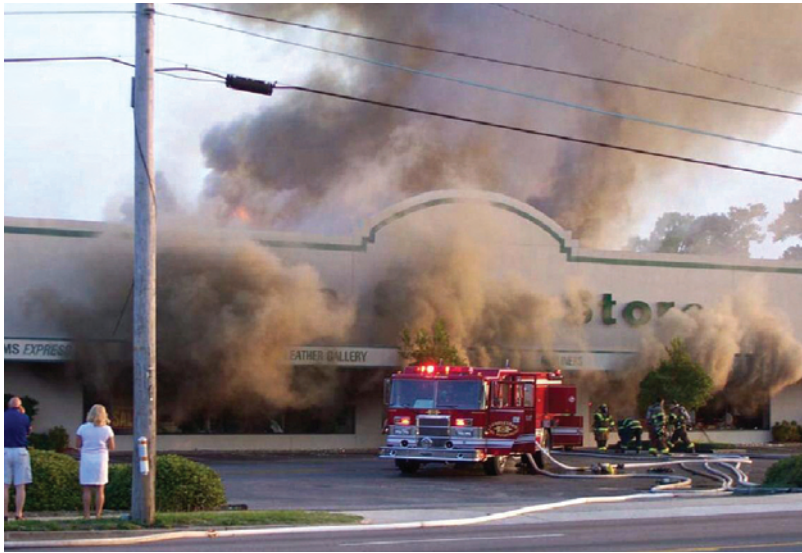
Photo 5: Shortly after the front windows of the building were removed in an effort to horizontally ventilate the building, the fire grew rapidly inside. Without adequate water supply for the hose lines inside, there was little hope of controlling the fire.
