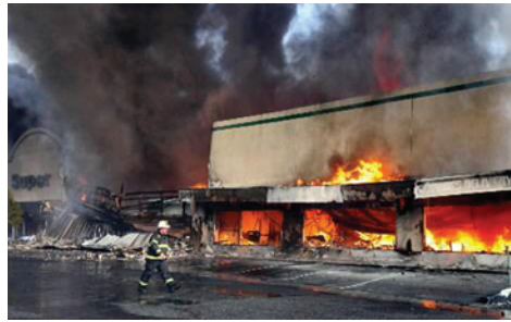
Photo 6: The building façade that created a parapet wall at the front of the building that prevented access for normal roof ventilation collapsed along with a major portion of the roof.
