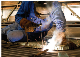
Photo 1: Shielded metal arc welding, down-flat welding position.
