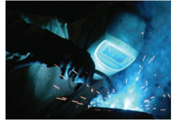
Photo 3: Flux-cored arc welding, down-flat welding position.
