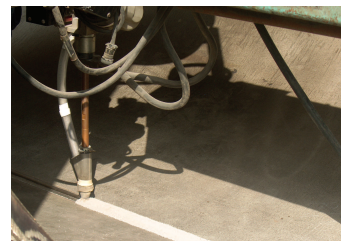
Photo 5: Submerged arc welding.
