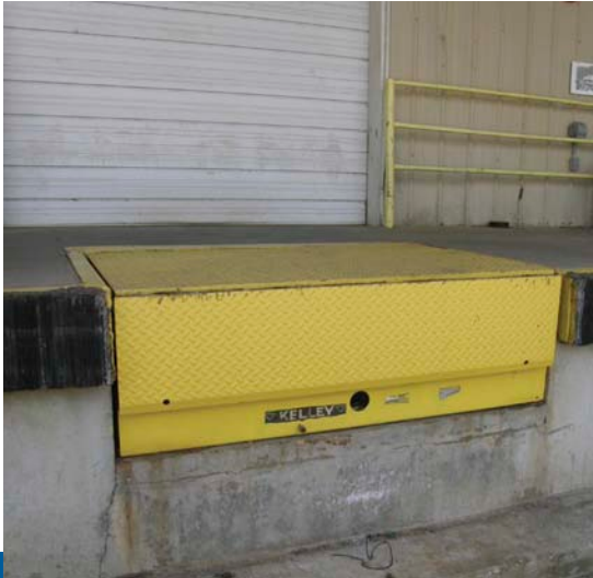
Photo 7 shows a dock leveler, which employers often fail to recognize as PRCS.
