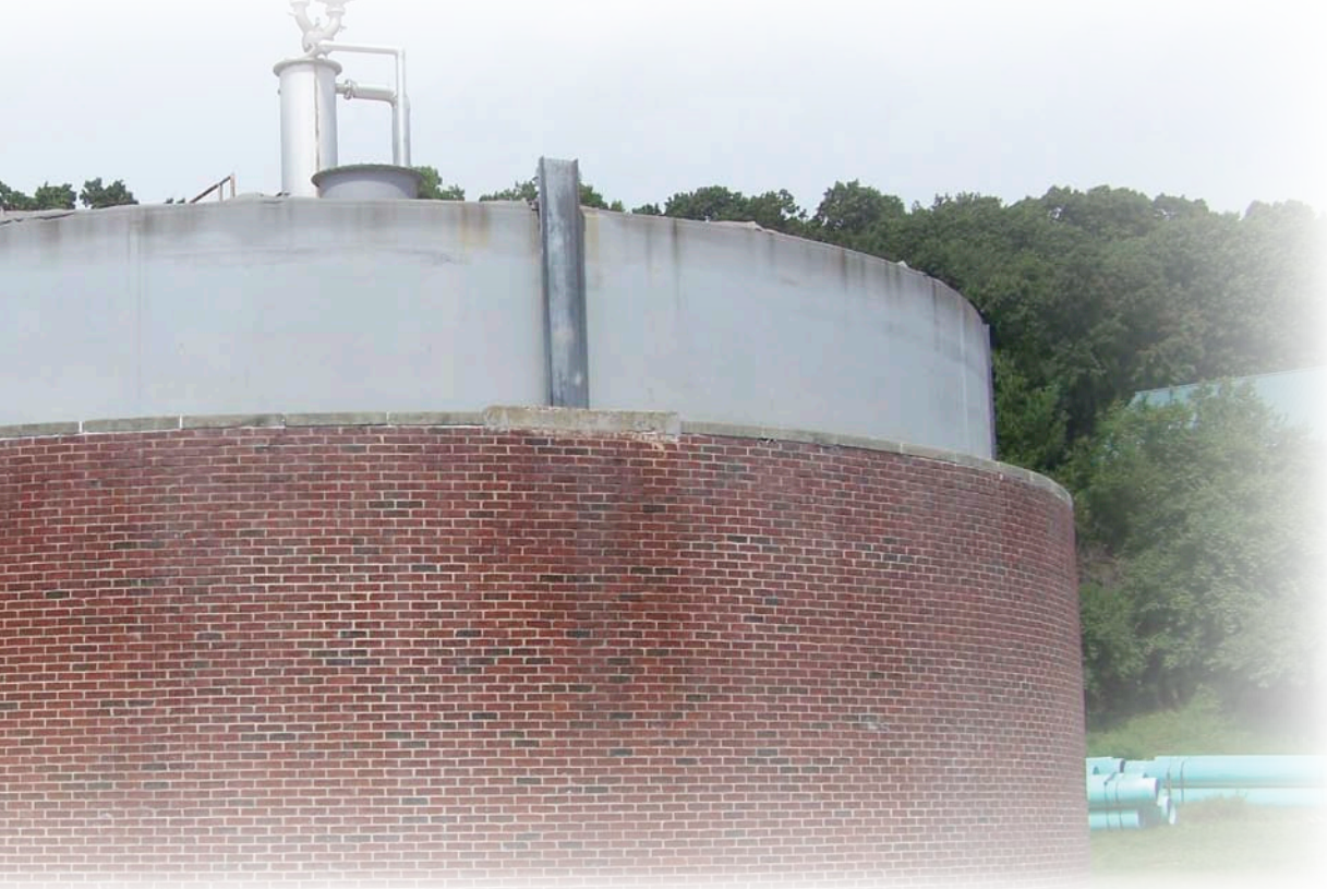
Photo 1: Typical anaerobic sludge digester building.
