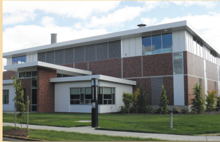
Photo 2: Increased window areas may create additional fall hazards during construction.
