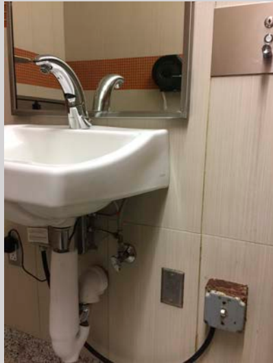
(Clockwise from top) Photo 3: A visual assessment of the cord depicting the plug and affixed manufacturer labeling and warnings, which should remain legible on the appliance. Photo 4: The result of a bathroom appliance installed without an electrical assessment; the switch is installed under a soap dispenser and the power plug is installed close to a sink, both of which create potential risk. Photo 5: An outlet tester can be used to test the outlet where an appliance will be placed, these tests should be documented to help formulate decisions.
