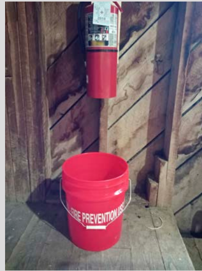
(Clockwise from top) Photo 1: Portable fire extinguishers and buckets for dousing fires should not be considered preventive measures because they are used once a fire is detected.
