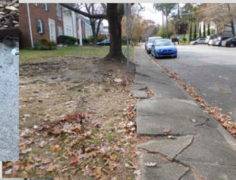
Photo 1 (left): Edging not flush with the walkway that allegedly caused a fall. Photo 2 (below): A sidewalk with major uplift from tree roots.
