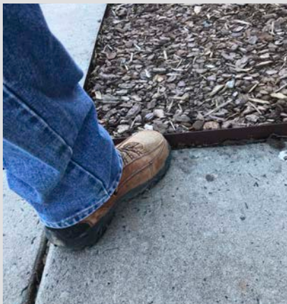
Photo 1 (left): Edging not flush with the walkway that allegedly caused a fall. Photo 2 (below): A sidewalk with major uplift from tree roots.
