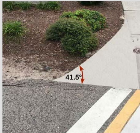
(Left to right) Photo 5: Concrete addition to eliminate 90° junction. Photo 6: Bent landscape edging due to high pedestrian traffic along desire line.
