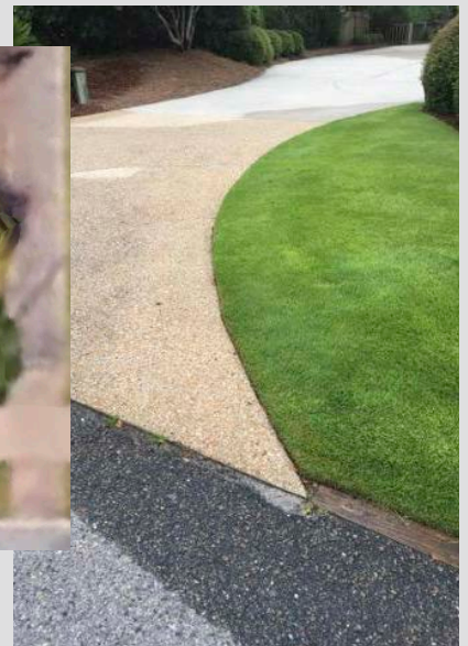
Photo 7 (above): Driveway radius of curvature with 10-ft diameter. Photo 8 (right): No edging along driveway.
