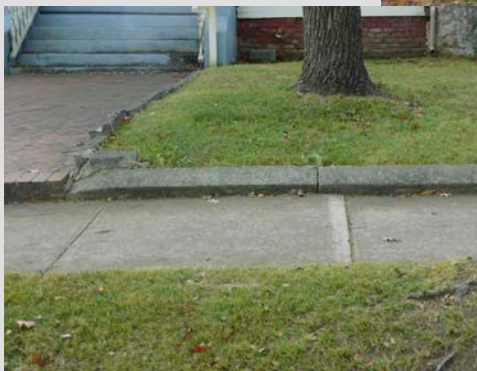
Photo 3 (above): Example of a beveled sidewalk because of uplift. Photo 4 (right): Campus desire path.
